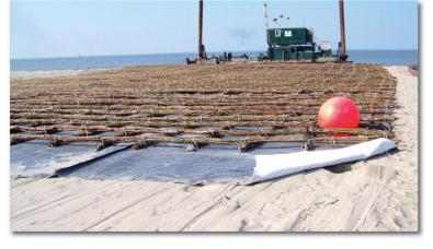
The solution for this dilemma has been found through the utilization of highly engineered, modern geotextiles and traditional fascines.
