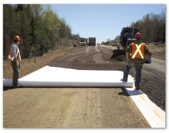
For a stretch of Hwy 62 south of Bancroft, the Ontario Ministry of Transportation, working with design engineering firm Golder Associates, sought a separation, reinforcement and drainage/filtration solution that punched nonwoven geotextile (Secutex®) – all in a single ma-
