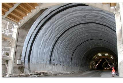
the overlapping seams must be 100% waterproof. Sealing experts and construction supervision teams test each seam for tightness
