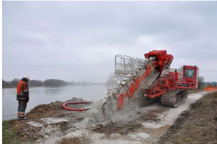
Figure 3.148: Machine used to mixed soil trenches using the dry method (figure from: DREAL CVL / DETL)
