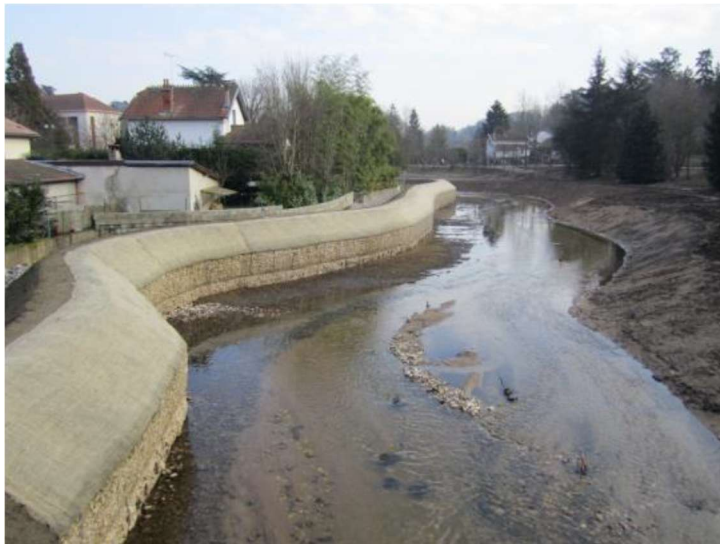
Figure 3.183 lope protection with 732 g/m 2 jute mesh fabric – immediately after installation (Photo Credit: CNR – Charbonnières)
