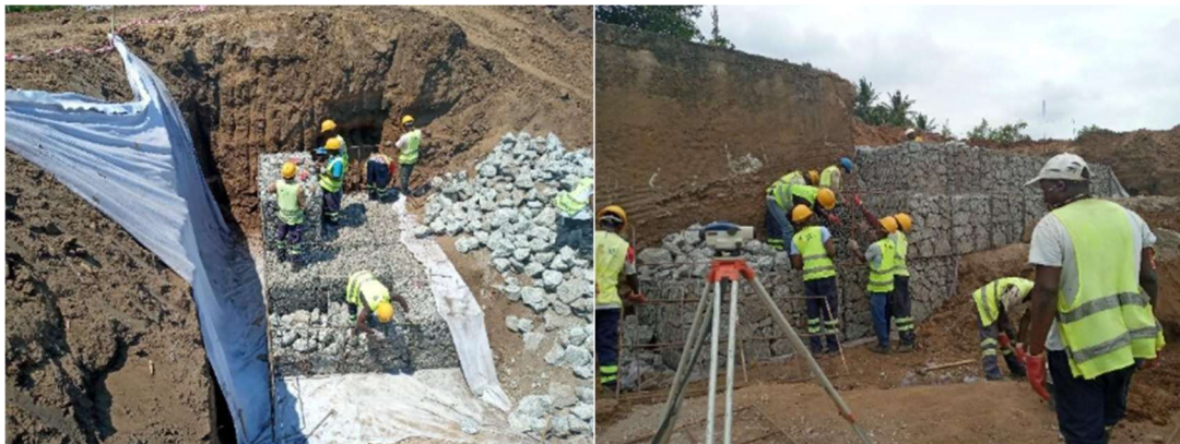
Figure 3.160 Construction of gabions wing Wall, river side
