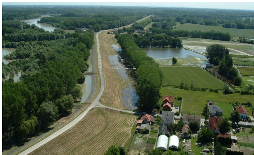
Figure 3.22 The investigated site
