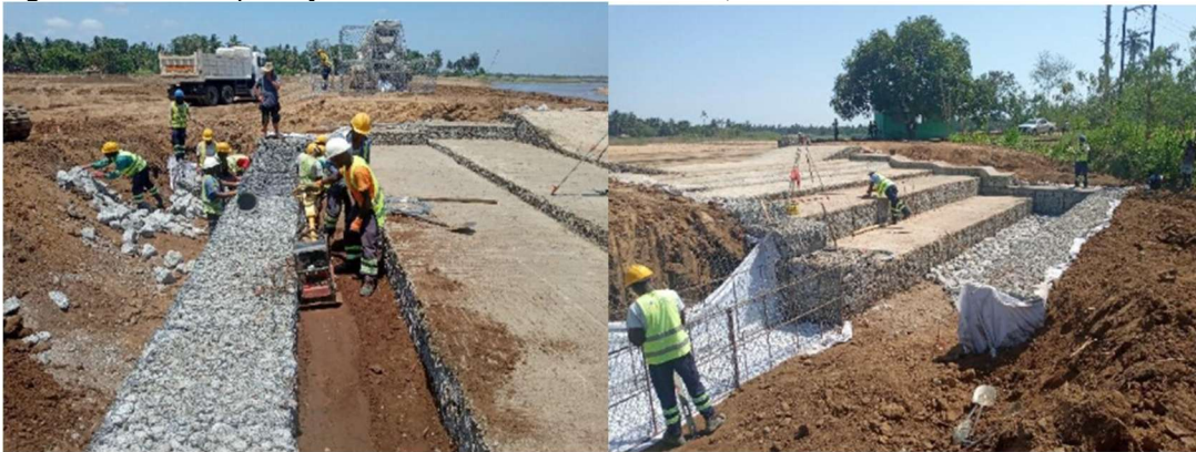
Figure 3.165 Execution of the cascade
