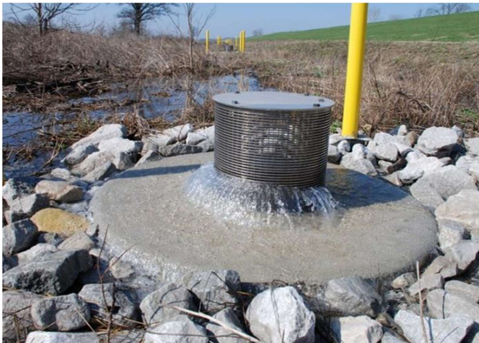
Figure 3.4 - Relief Wells flowing during high water 2016 in Arkansas
