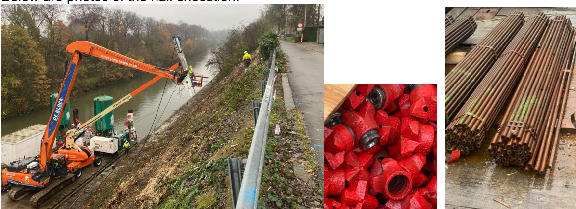
Figure 3.203 Photos of the execution of installing nails
