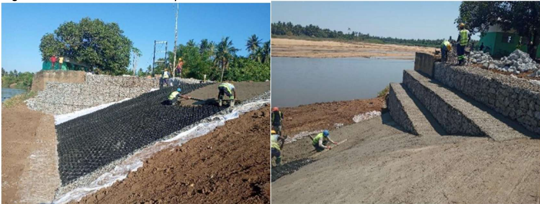
Figure 3.162 Execution of spillway on the river side.
