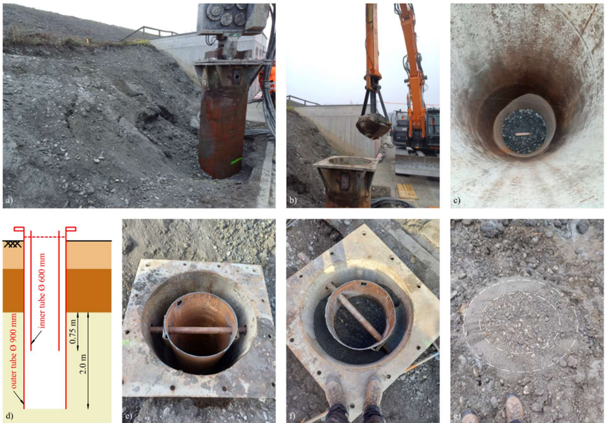
Figure 3.152: Construction of filter gravel columns: a) Vibrating the outer pipe into place; b) & c) Excavation with clamshell bucket; d) & e) Installation of the inner pipe; f) Backfilling with filter gravel; g) Finished filter gravel column.
