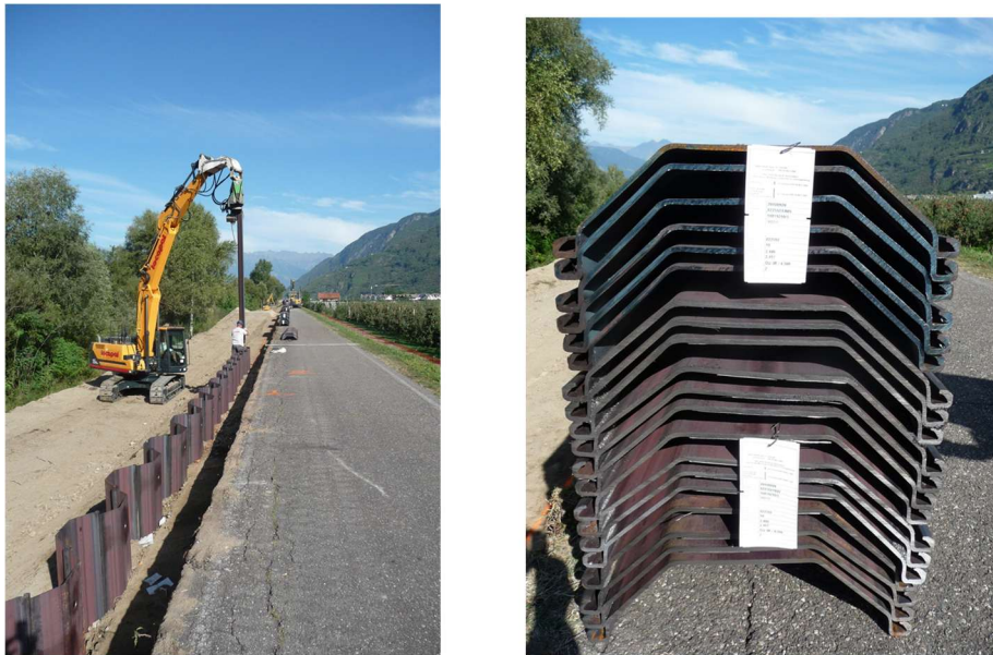
Figure 3.137 Installation of sheet pile walls.
