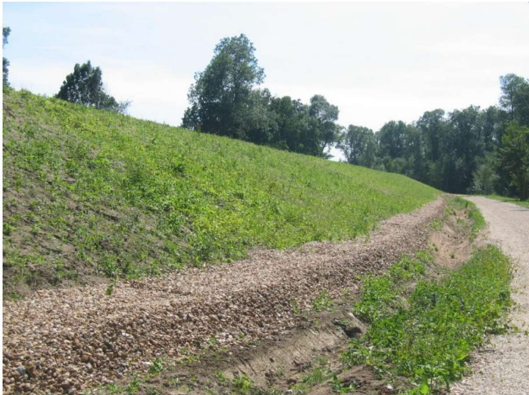
Figure 3.217 Drainage berm on a Loire dike: the granular part stands out clearly from the body of the dike. The ditch located between the toe of the slope and the maintenance track serves as the collection system for drainage water. There is no specific surface protection on this system, as the manager wishes to keep it visible during periods of operation (Photo credit: DREAL Centre Val de Loire).
