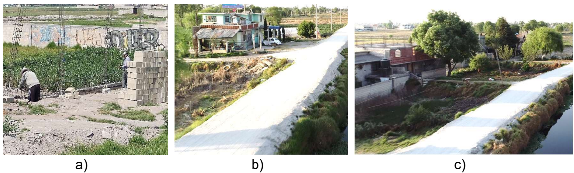
Figure 3.59 Identification of construction and settlements close to the levee. Source: a) Robaldi-Vazquez (2023b). b, c) Jiménez Gonzáles (2019)
