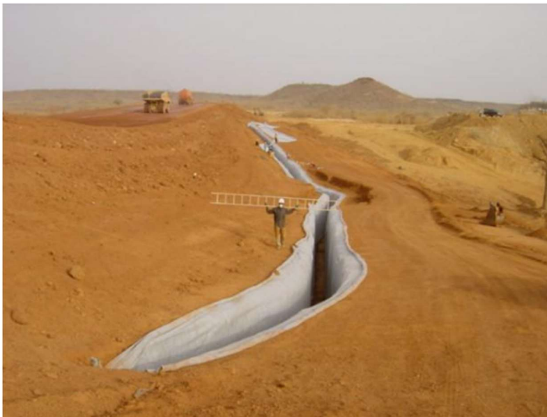
Figure 3.218 Construction of a drainage trench at the toe of the dike on the protected side. Note: Safety instructions for personnel working on site are specific to each country; in this case, the Samira Dike in Niger (sheet C3-6). (Photo credit: Olivier Artières)
