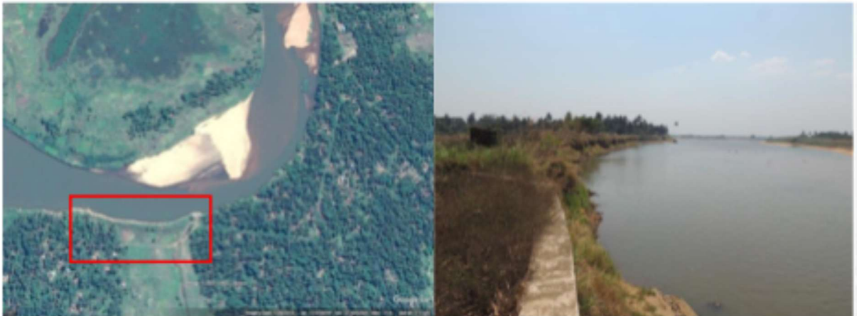
Figure 3.78 The stretch downstream of Intabo pumping station in September 2013 and November 2014
