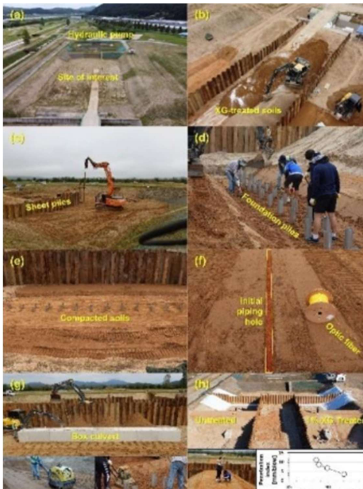
Figure 3.157: Construction process of the full-scale levee
