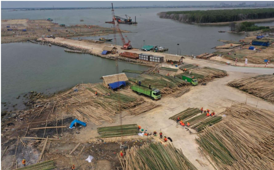
Figure 3.199. Construction of embankment improved by bamboo-mattress reinforcement.
