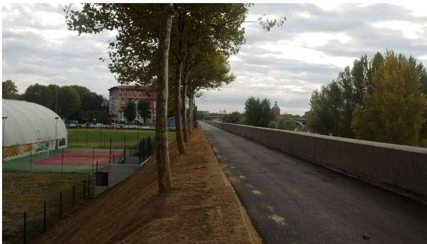
Figure 3.38 after installation of the coconut mat and seeding (courtesy: DDT31)
