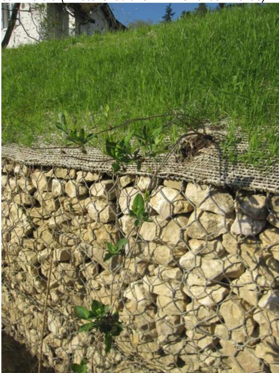
Figure 3.187 Gabion–earth dike at Charbonnières – geogrid + 732 g/m 2 jute geotextile + seeding + climbing plants – side view (Photo Credit: CNR – Charbonnières)
