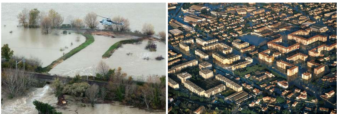
Figure 3.85 Flooding of the Rhône delta in December 2003 (© SDIS13 and J. Roche)
