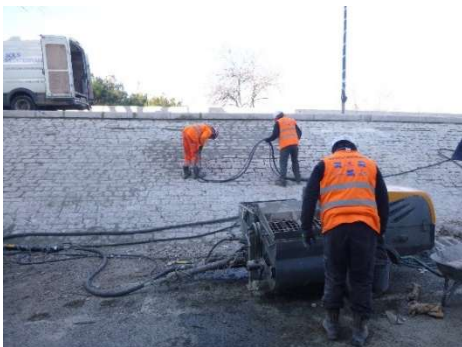
Figure 3.193 Site installing new joints - Injection pump and air gun (Photo credit: BRL i )
