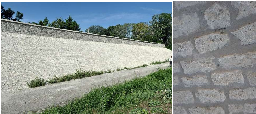
Figure 3.194 Photograph of a renovated facing (Photo credit: BRL i )
