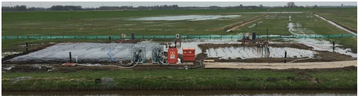
Figure 3.98 Overview of the area
