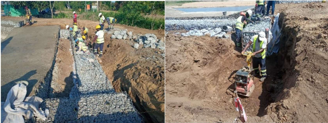
Figure 3.164 The spillway crest and works on the cascade, land side
