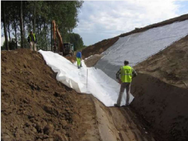
Figure 3.216 Construction of a drainage layer at the toe of the slope on the protected side. The excavation shape was created using an excavator bucket. In the foreground, the installation of a geosynthetic filter; in the background, the drainage gravel placed on the geotextile, awaiting coverage by the filter and a layer of topsoil – Amboise (37). The excavation depth does not require shoring, and the slopes are stable in the short term (Photo credit: DREAL Centre Val de Loire).
