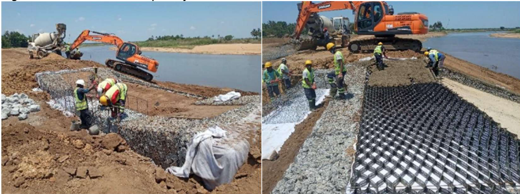
Figure 3.163 Execution of the spillway crest (access for maintenance)
