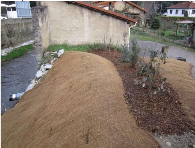
Figure 3.185 Protection of a small embankment slope using 900 g/m 2 coconut geotextile – immediately after installation (Photo Credit: CNR – Charbonnières)
