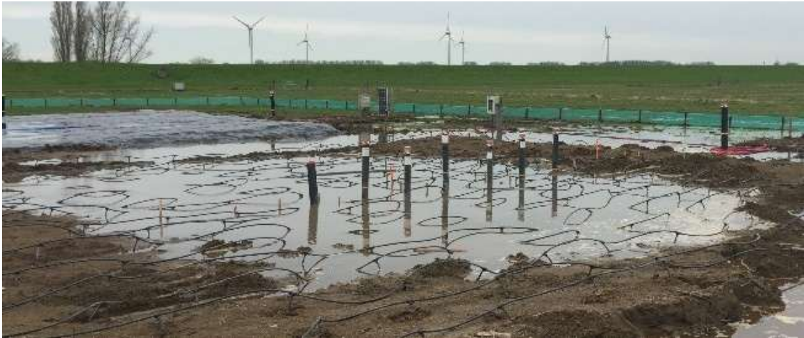
Figure 3.102 Beadrain-S section with monitoring equipment (after some days of consolidation).
