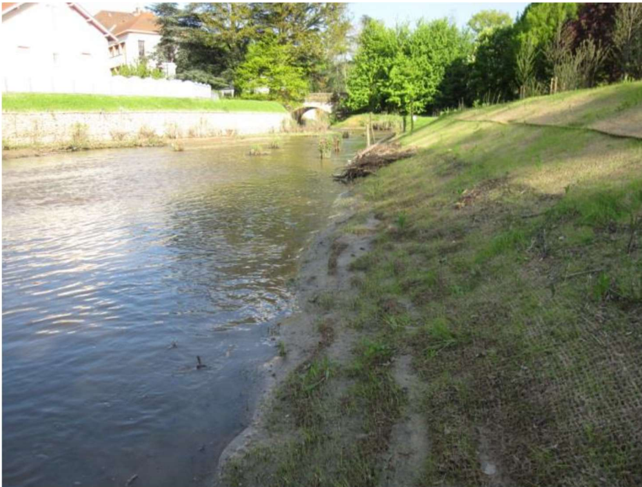
Figure 3.186 900 g/m 2 coconut geotextile on a section of dike exposed to the watercourse – flood debris still visible (Photo Credit: CNR – Charbonnières)
