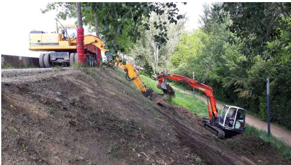
Figure 3.34 stripping of the slope (courtesy: GTM; DOE)
