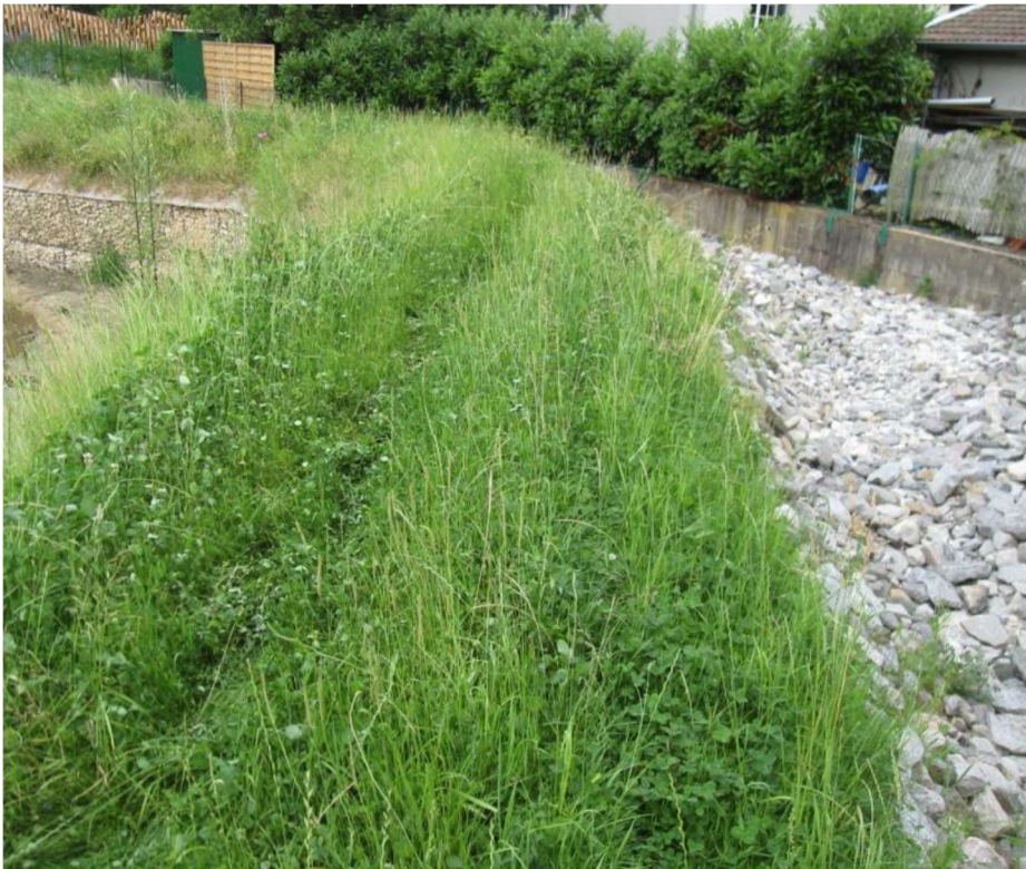
Figure 3.188 Gabion–earth dike at Charbonnières – geogrid + 732 g/m 2 jute geotextile + seeding – top view (Photo Credit: CNR – Charbonnières)
