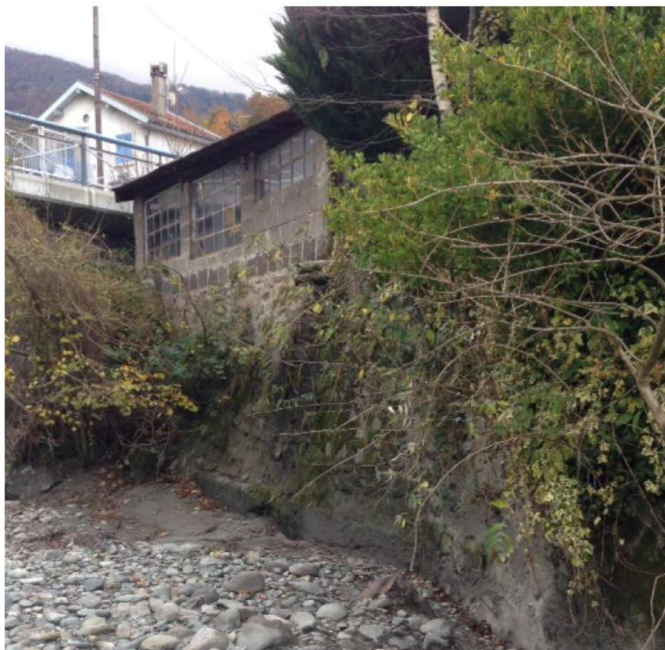
Figure 3.168 Situation before Consolidation - La Romanche in St Pierre de Mésage, Isère (Photo credit: ARTELIA)
