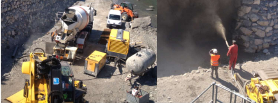
Figure 3.173 Shotcrete work site (Photo credit: ARTELIA)
