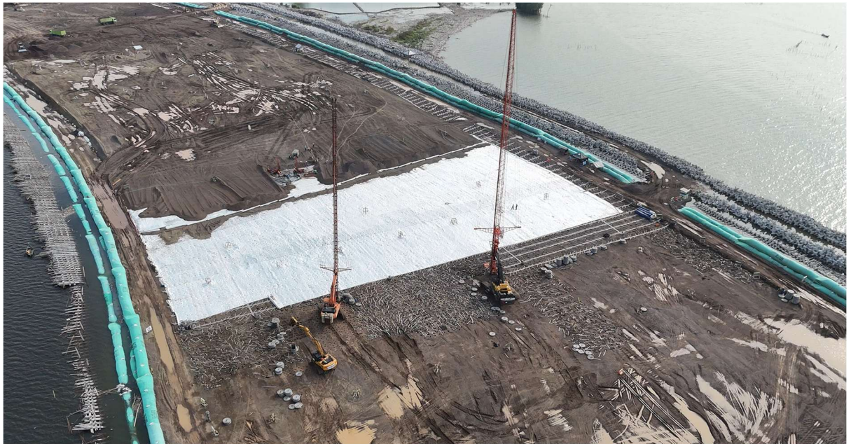
Figure 3.109. Installation of high-strength woven geotextile and PVD after installation of the bamboo-matress reinforced fill.
