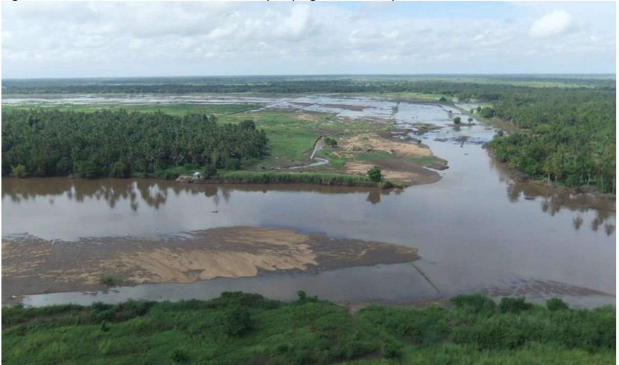
Figure 3.79 The aftermaths of 2015 floods in Intabo, showing the major breach.
