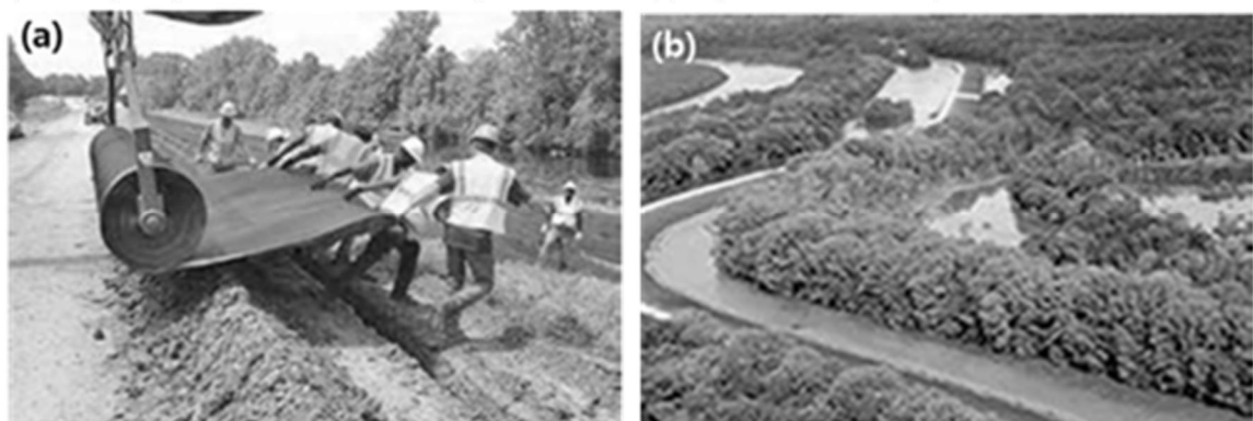
Figure 3.47 (a) Installation process of geosynthetics [8]; (b) Example after completed installation.[8]
