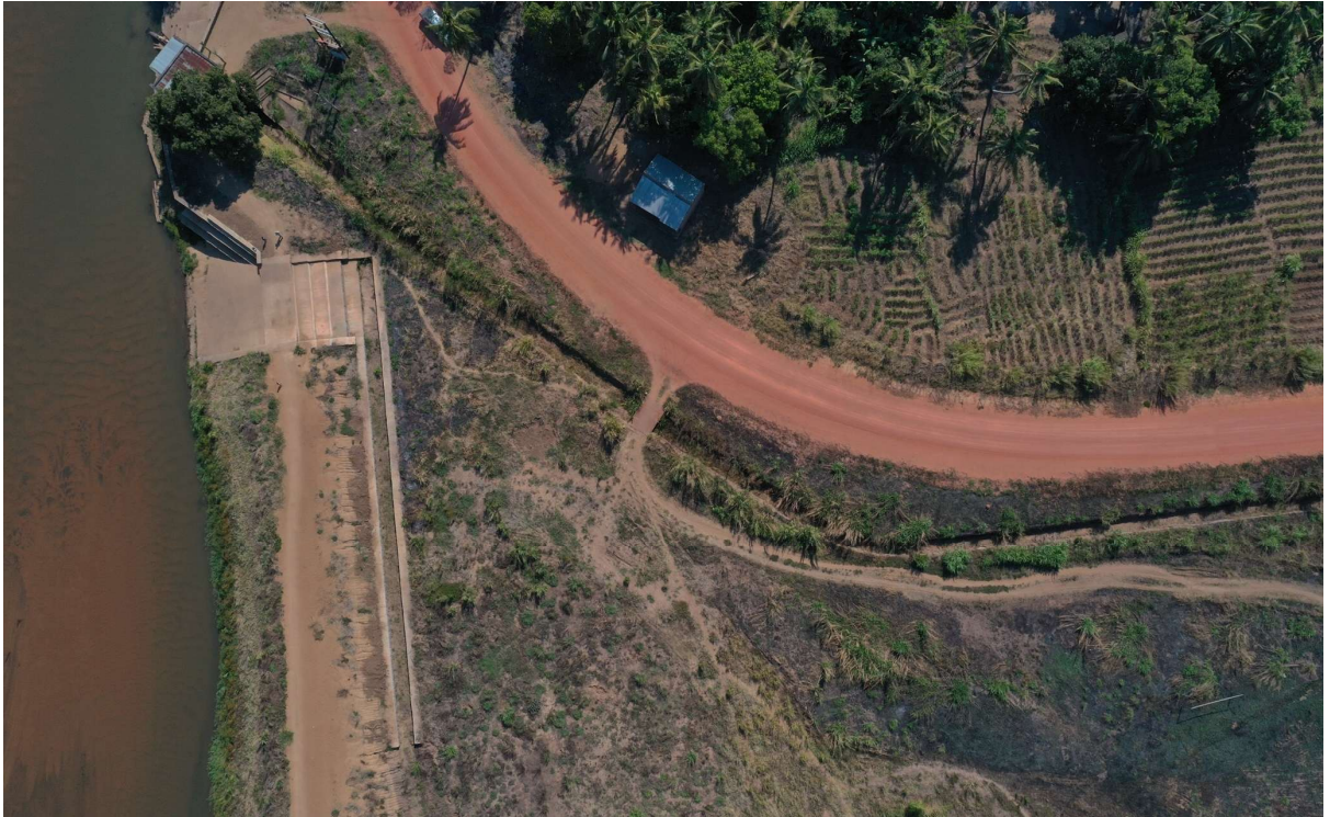
Figure 3.84 Birds eye view of the Intabo Spillway after the 2022 floods
