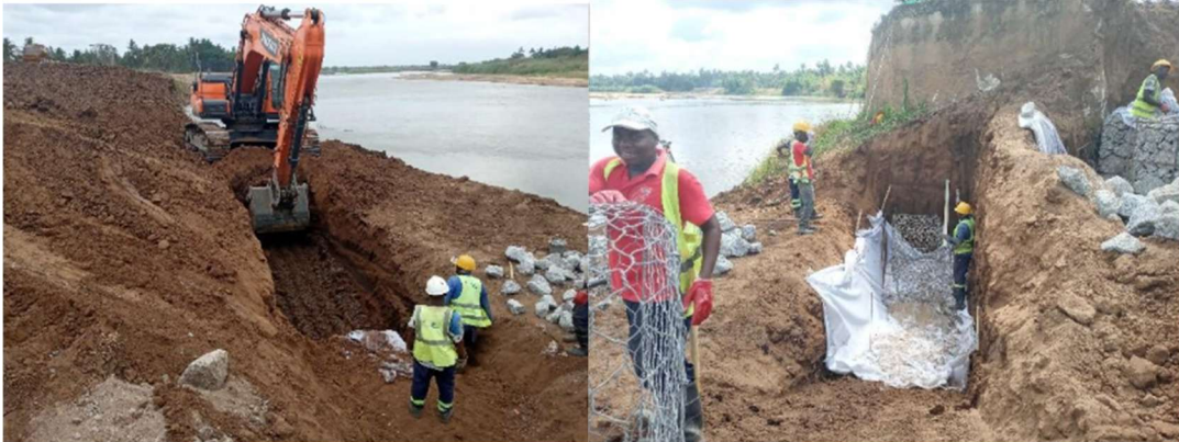
Figure 3.161 Execution of toe protection on the river side
