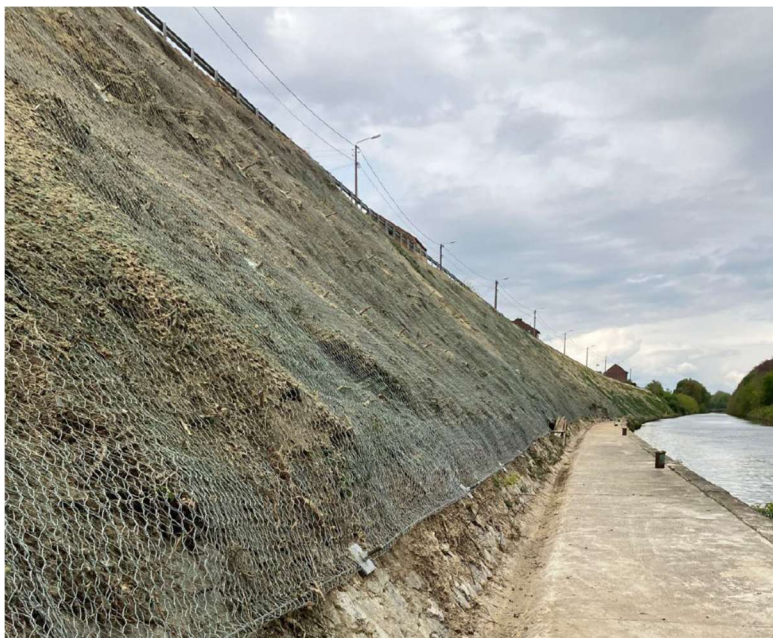
Figure 3.204 Picture of the slope after reinforcement, including steel wire mesh
