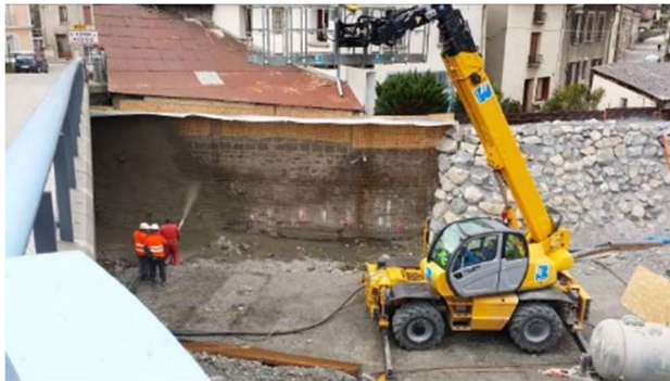
Figure 3.169 Example of dry spraying - La Romanche in St Pierre de Mésage, Isère (Photo credit: ARTELIA)
