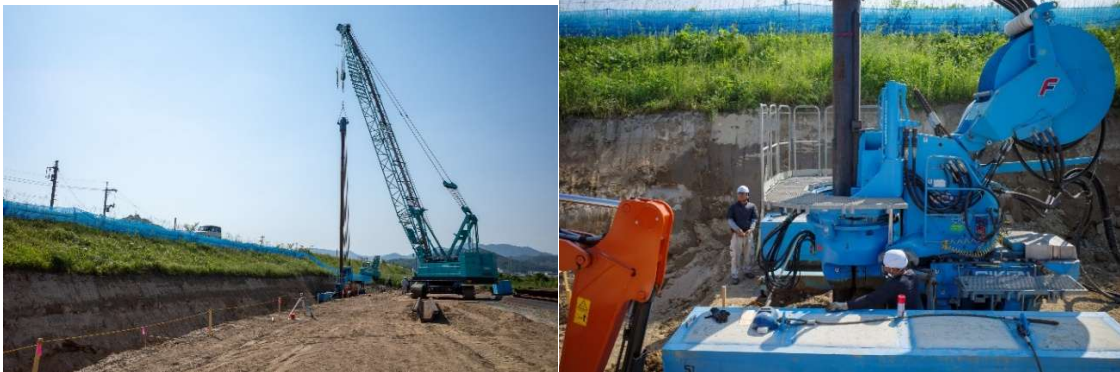
Figure 3.151 Left: Construction of sheet piles, Right: Construction machinery for a sheet pile
