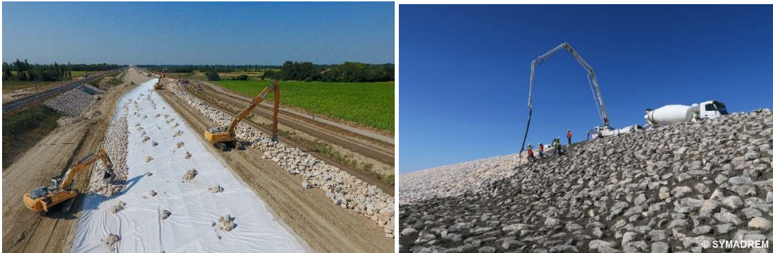
Figure 3.177 Stage 3 : rip rap on second geotextile (left) – Stage 4 concreting of rip rap (right)
