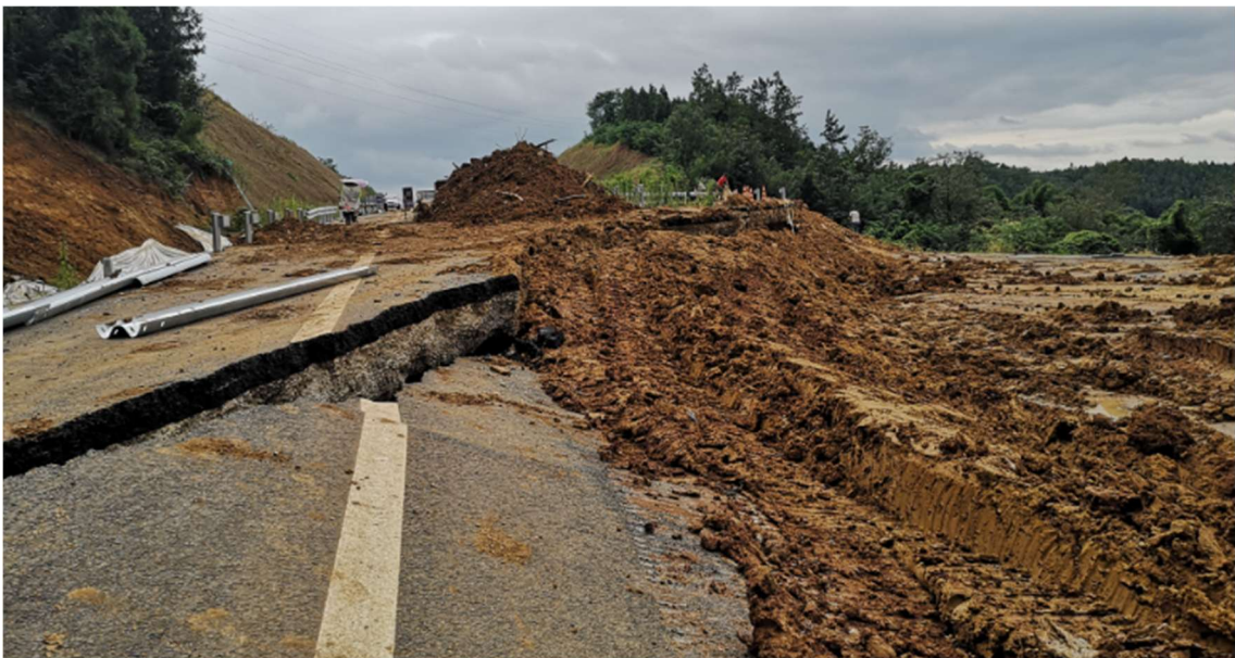
Figure 3.123 Embankment at the Long Downhill Section of the Route
