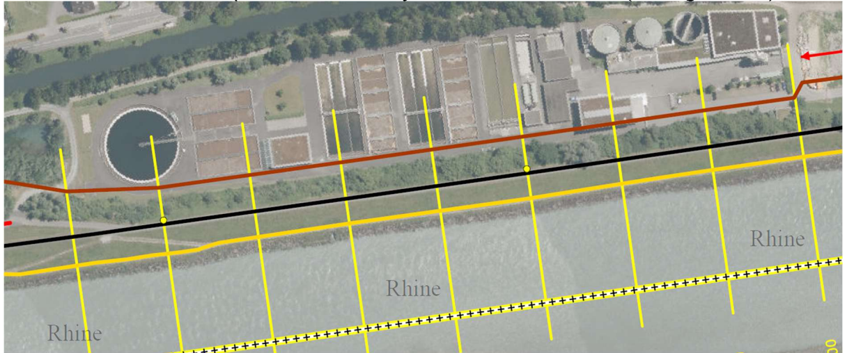
Figure 3.29: Remediation section directly adjacent to a wastewater treatment plant before remediation measures (yellow lines every 50 m) (source internal project documentation, Ingenieurbüro Sprenger & Steiner)
